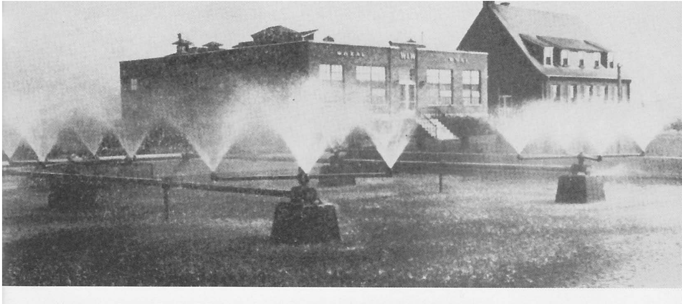
“The Fountain” –Cooling spray pond at 500 kW WLW (1932)
