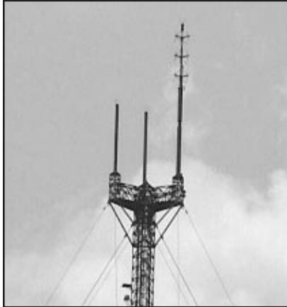
Figure 1. Photo of the Madison Community Tower, as seen when facing west. The current antenna configuration shows WMSN-TV on the left, WKOW-TV/WKOW-DT in the center, and WISC-TV stacked on top of WHA-TV on the right.
