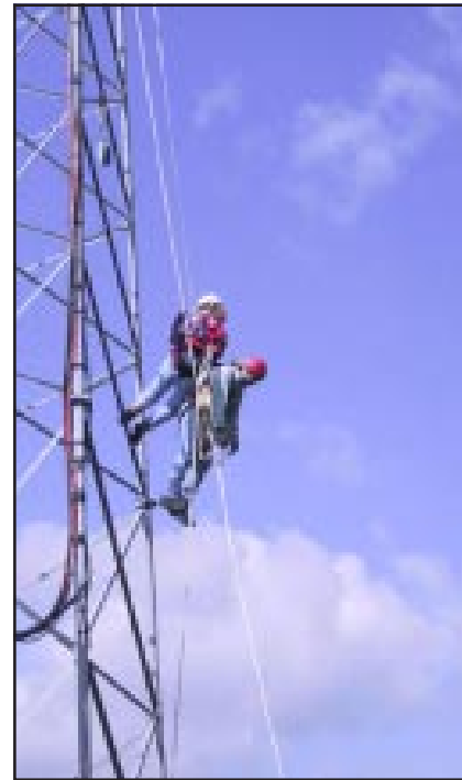
Figure 6. I'm using a Fisk descender to lower an injured technician to the ground. Photo by ComTrain.
