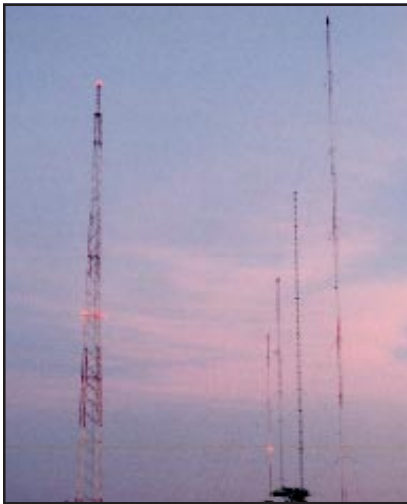
Figure 1. Towers lit at night to warn airplanes.
