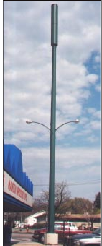
Figure 8. Light pole monopole tower for cellular applications.
