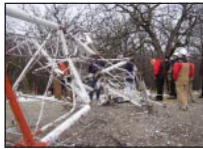
Figure 8. Workers observe the twisted steel.
