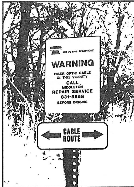
Figure 1. A typical sign identifying the location of an underground fiber-optic cable.
