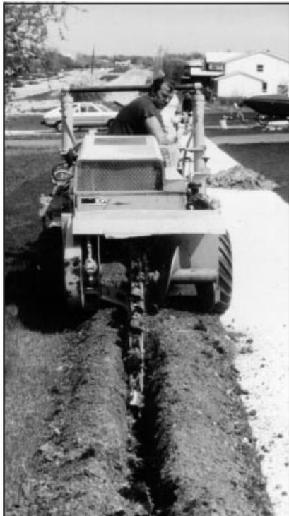
**Figure 1.** Trenching for cable television trunk cable, Madison, 1977. This photo shows the installation of trunk cable along the south side of Raymond Road just west of Frisch Road. Note that Raymond had not been paved west of Frisch at the time this photo was taken.
