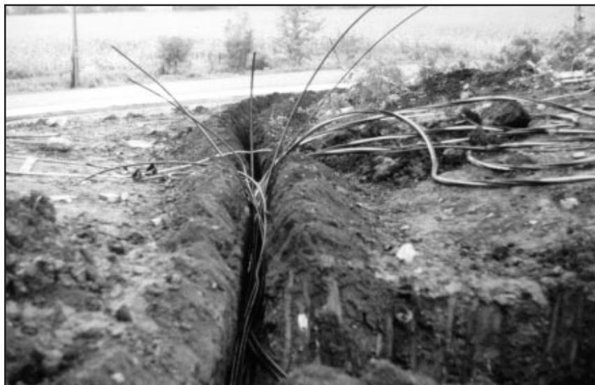
**Figure 2.** Direct-burial trench, Fitchburg, 1980. This is a "joint trench" containing facilities owned by three companies: electric power (MGE), telephone (TDS), and cable television (Fitchburg Cable Communications, now Marcus).
