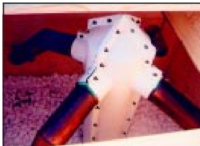
Figure 5. Jampro FM transmit antenna.
