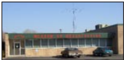
Figure 1. Pavek Museum is in the St. Louis Park suburb of Minneapolis.
