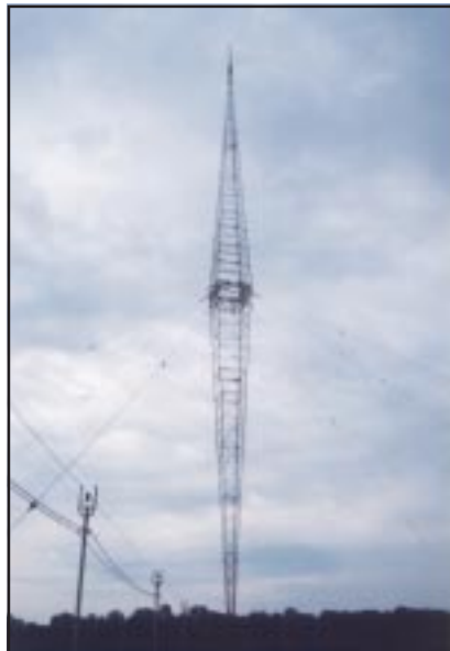
Figure 1. The pole at the top of the WSM-AM antenna tower holds a turnstile FM antenna for the now defunct WSM-FM 100.1 MHz station. The functionality of the open air transmission lines (lower left) have been replaced by underground transmission lines.
